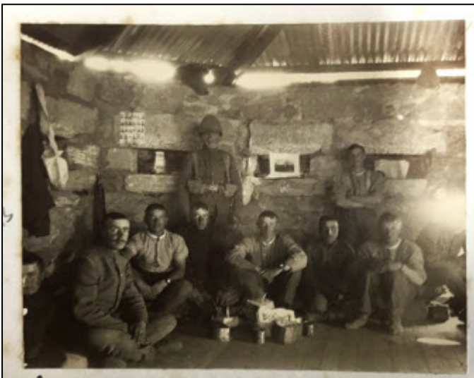
Below: 3 Bttn blockhouse
